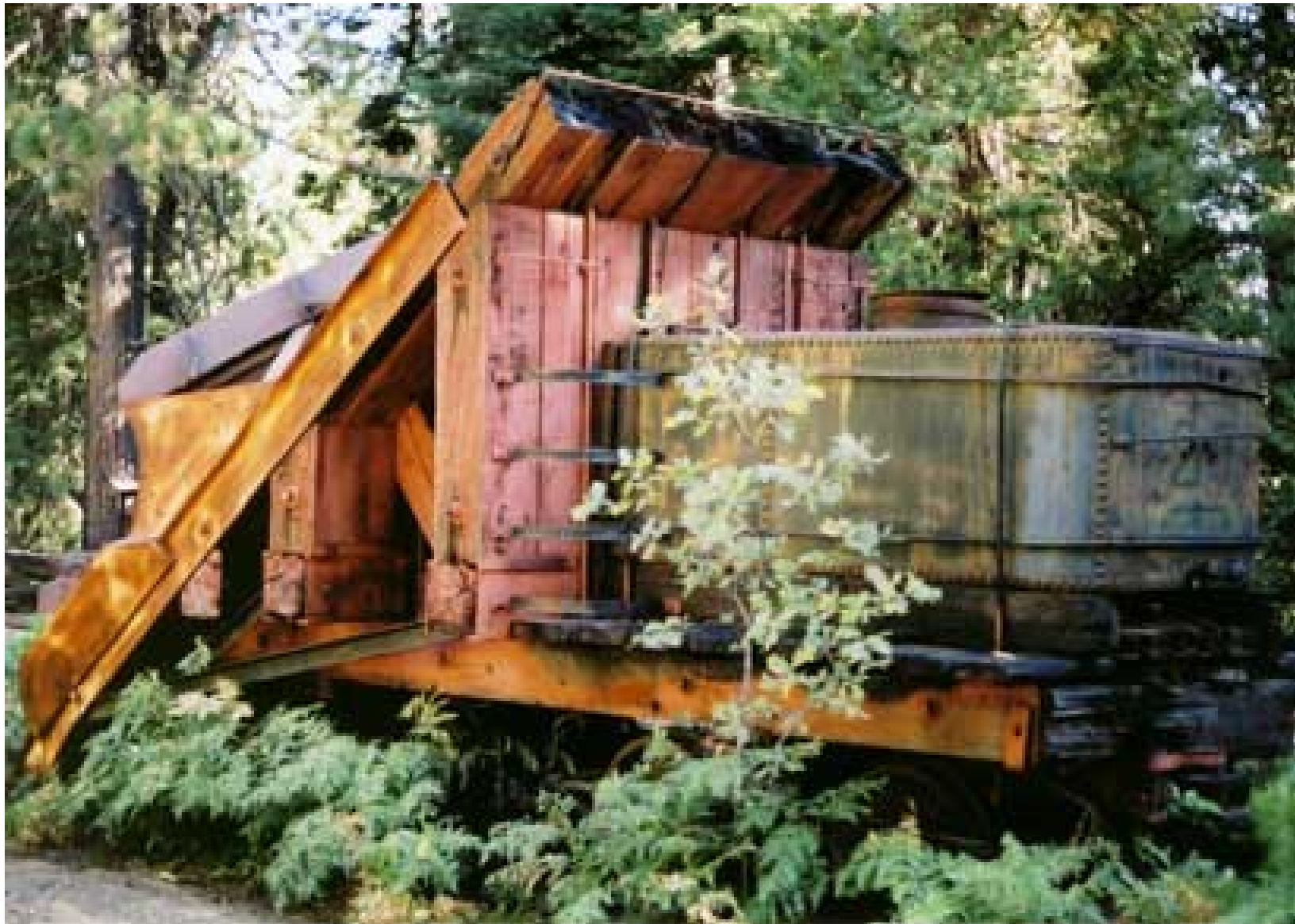
Look at the end of beams on the plow – black color with grain. Paint missing on the rest of the wood. Stains everywhere.
